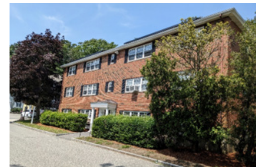
Powder House Lane (29 units in 2 buildings on 2 acres- density of 15 units per acre)
