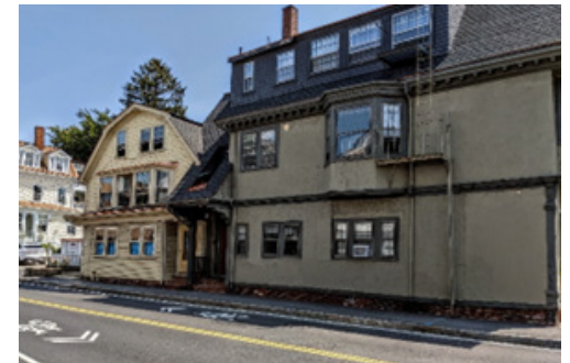
1-3 School Street (13 units on .14 acres- density of 92 units per acre)
